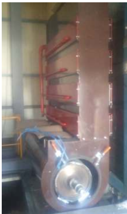
Steel Roll Washing Tanks
